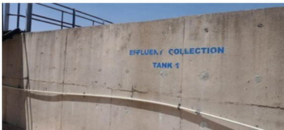
A poultry processing plant has a well-functioning effluent treatment system
